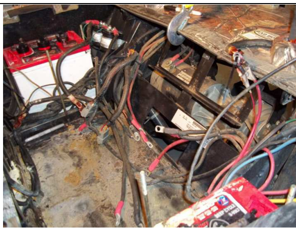
Controllers removed, brush any rust and coat of paint
